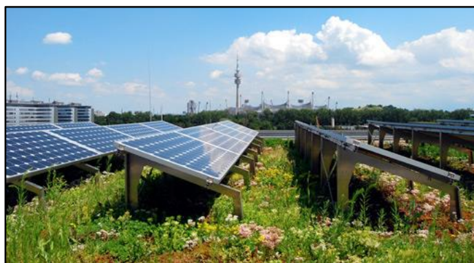
Figure 32: Green roof with PV panels
