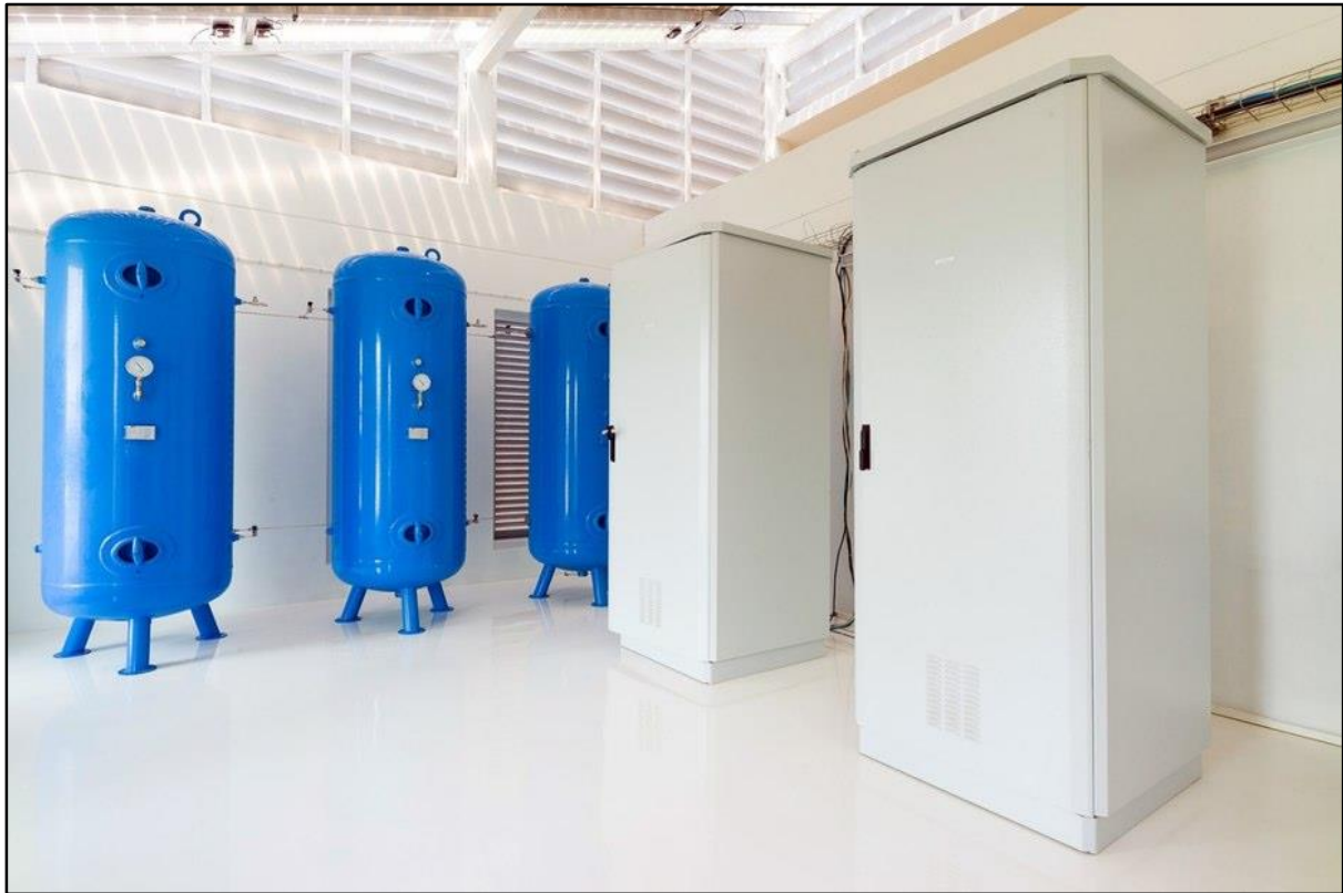
Figure 13: Hydrogen production and storage at the Phi Suea House project
